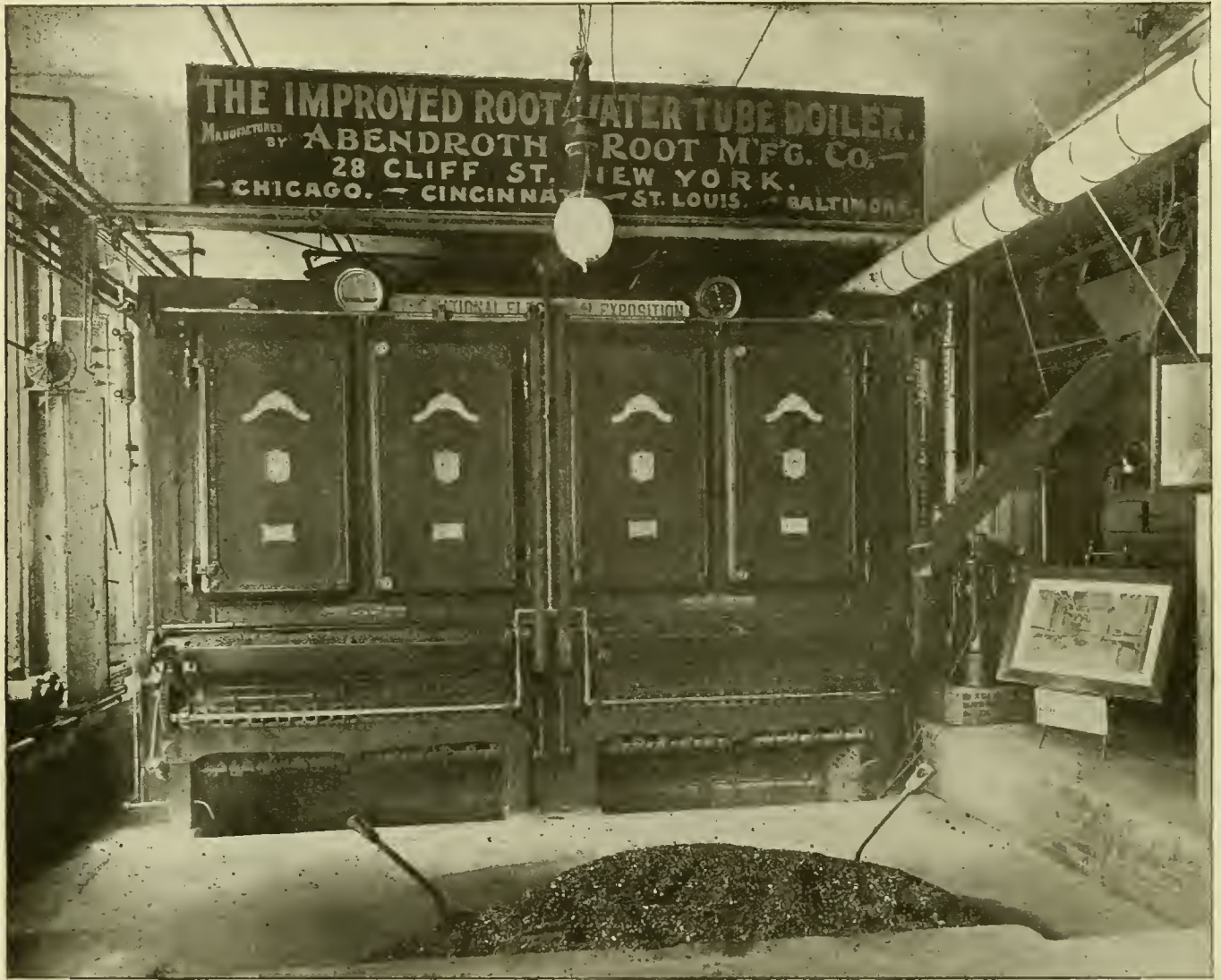
Exhibit of Root's Improved Steam Boiler at the National Electrical Exposition.
